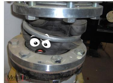
The rubber joint is unmatched for vibration isolation. If properly installed, a rubber joint can greatly reduce equipment nozzle loads. Its resilience allows it to be installed in many different systems under a range of temperatures, pressures and media. What could possibly go wrong?
