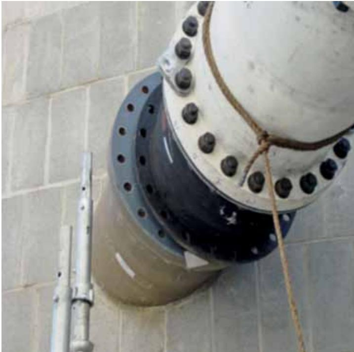
Figure 3. Large pipe misalignment
