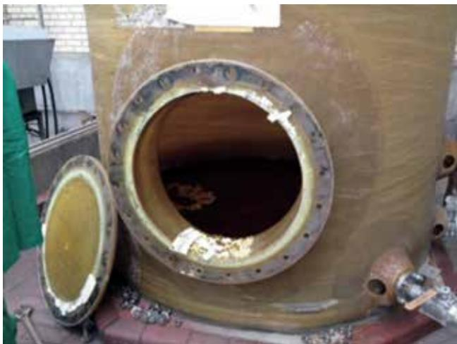
Image 1. Manway of an HF acid re-boiler
