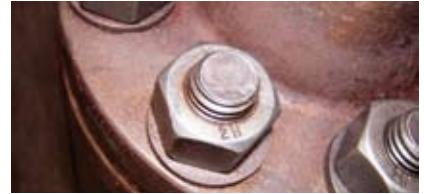
Figure 2. ASTM Grade A194 H2 Nut
