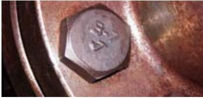
Figure 1. ASTM Grade A193 B7 Bolt
