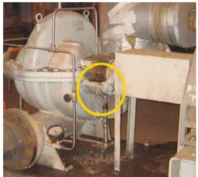
**Figure 2.** Packed pump with excessive flush pressure.
