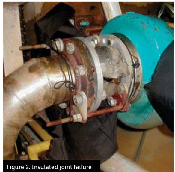
Figure 2. Insulated joint failure
