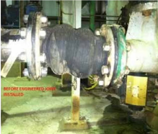
IMAGE 2: Example of misalignment over time. The joint in the picture is compensating for lateral offset.
