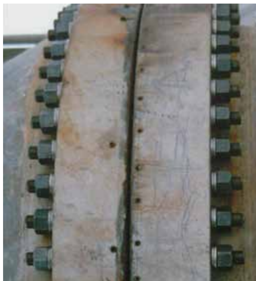
Image 1. The use of conical washer springs between the bolts and gasket flange ( Images courtesy of the author )
