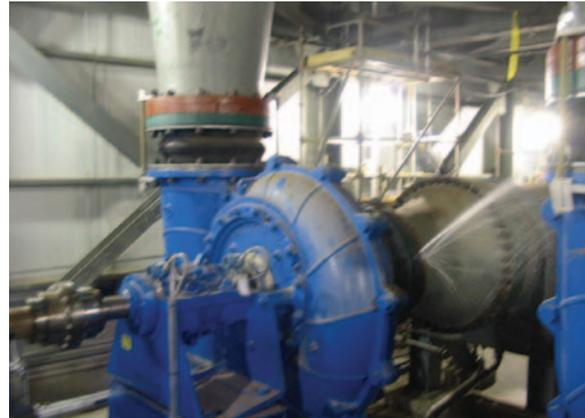
**Figure 1.** Newly installed expansion joint adjacent to slurry pump
