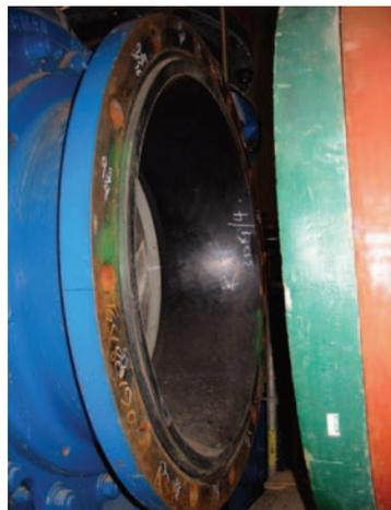
**Figure 2.** Raised rubber face on pump flange
