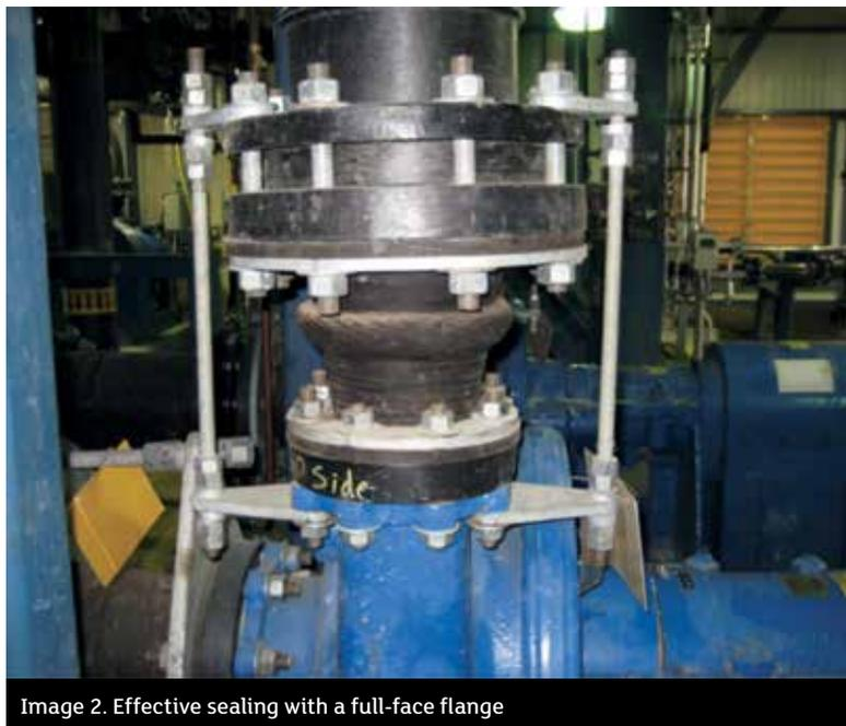
Image 2. Effective sealing with a full-face flange
