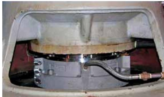
Image 4. Split seal installation— influent pump with a 15-inch shaft
