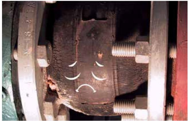
IMAGE 5: Hard-boiled expansion joint
