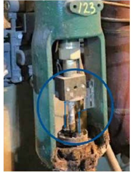
IMAGE 5: Axial clearance example needing radial clearance as guide
