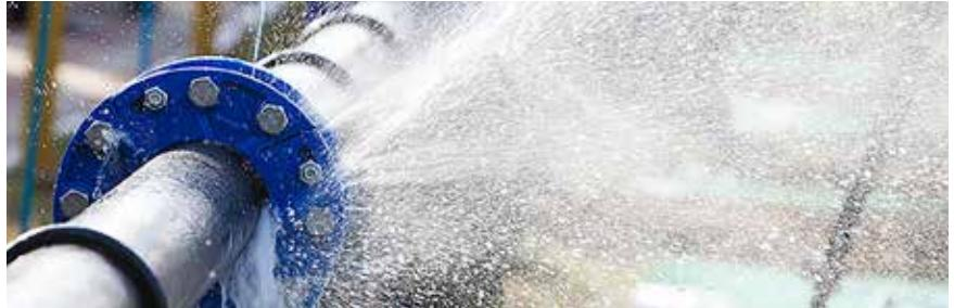
IMAGE 1: Improper gasket material selection and installation can lead to leaks (Image courtesy of Triangle Fluid Controls)
