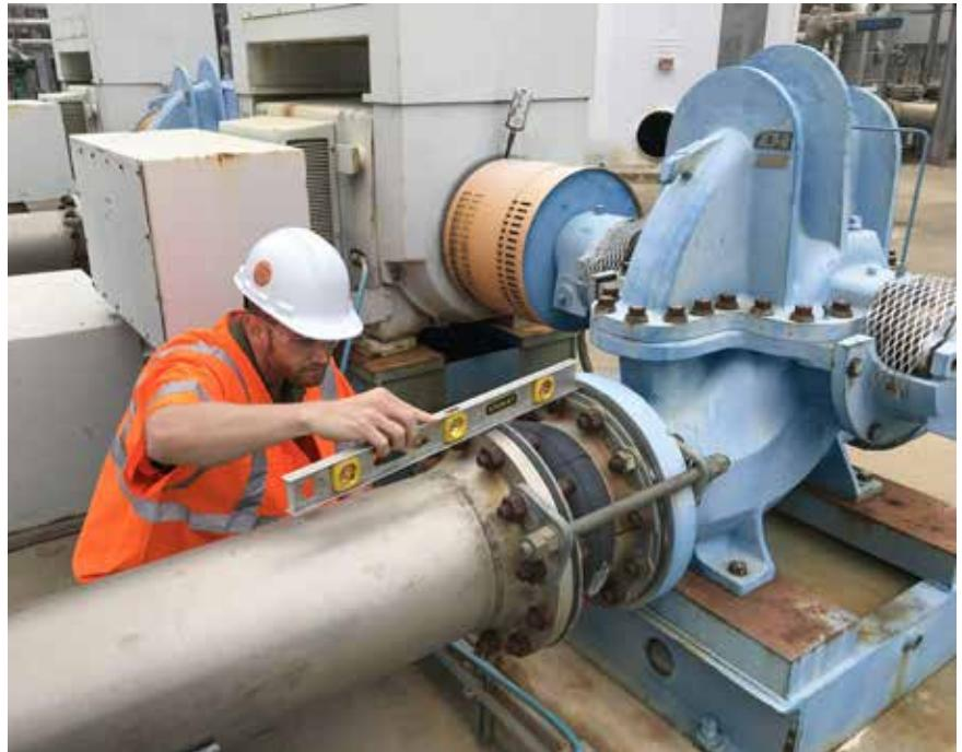
IMAGE 1: User conducting an expansion joint survey (Images courtesy of Proco Products)
