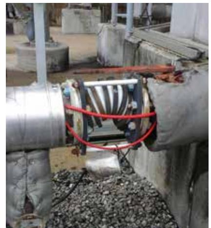
IMAGE 2: Faulty expansion joint installation
